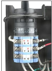
**Figure 16.** Motor power and direction switch.
